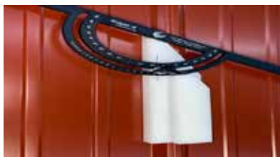
Ridge -L9. Mark your 9" o/c panels consistently. Degrees or pitch for gables, valleys or as needed.
