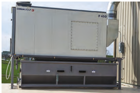
4 yd. Iron Bull Hopper designed for a F450 Comia Dust Collector
